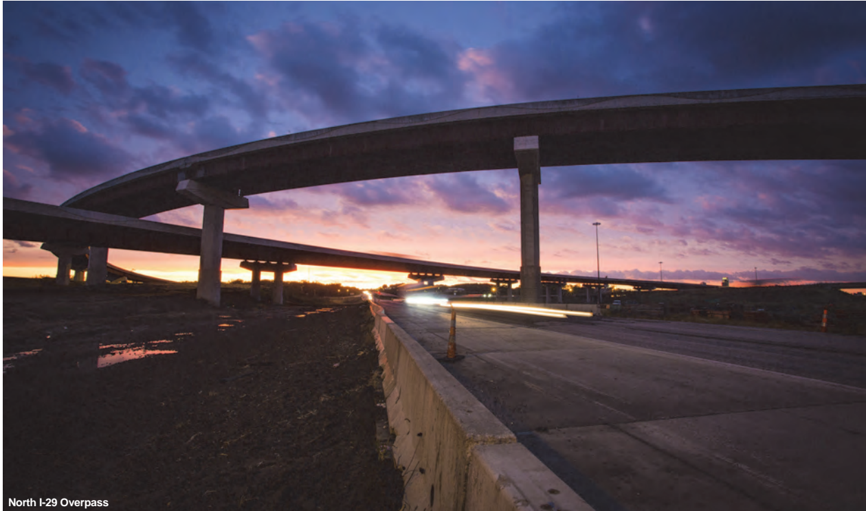
North I-29 Overpass
