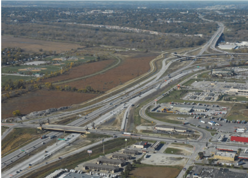
I-80/I-29 Dual, Divided Freeway construction east of the West System Interchange
